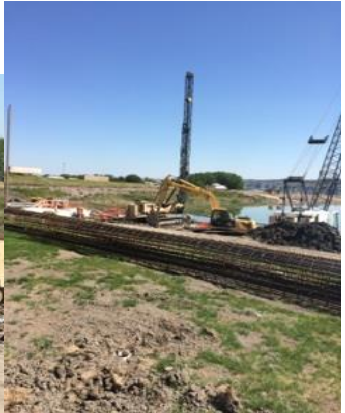
Drilling holes for concrete and rebar to anchor the hill side at Cedar Shores.
