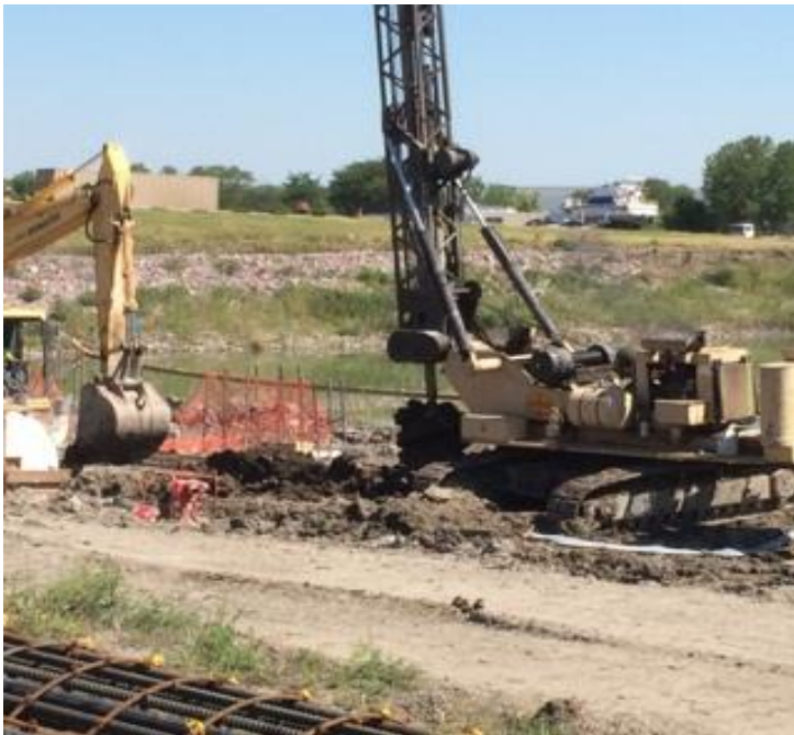
Drilling holes for concrete and rebar to anchor the hill side at Cedar Shores.
